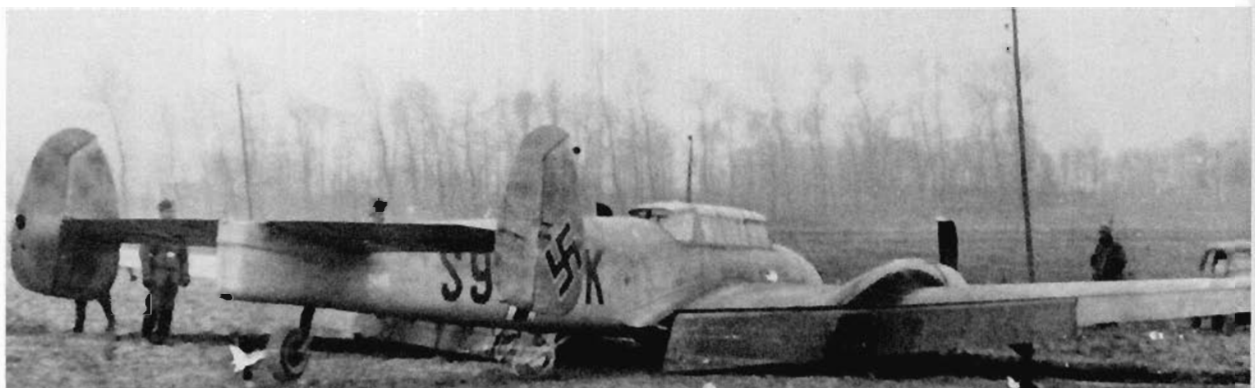
ABOVE AND LEFT: Uffz. Artez' Bf 110 D, S9+LK, of 2./Erprobungsgruppe 210 photographed after a forced-landing on 21 March 1941, following a night bombing attack. Camouflage was still 71/02/65 with a thin spray of 02 over the camouflage of the fuselage and engines. The extended tail cone housed a dinghy. (J.Vasco)
