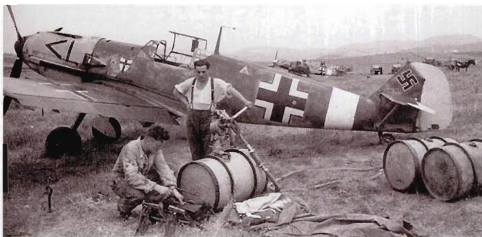
ABOVE: Seen amidst terrain for which its 71/02/65 camouflage had never been intended, a Bf 109 E undergoes an engine change in the open at a Libyan airfield. The unexpected drawing of the Luftwaffe into the Middle East conflict, launched by Italy, produced such anomalies until a range of suitable tropical camouflage colours could be hastily brought into production. The extensive mottling on the sides of the fuselage date the photograph to 1941. (D. Vincent)
