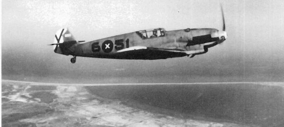
ABOVE AND RIGHT: Two photographs of Bf 109 D-1, 6051, finished in 62/65 colouring. However, close examination shows the original 70/71 camouflage beneath the thin 62 coating. The darker segments on the wings appear to be part of the original colours, retained as a rudimentary disruptive pattern, the section near the wing root being identical, though a larger segment appears to have been left inboard of the disc marking. The spinner was white, as were the six kill markings shown on the fin. The latter were those of its regular pilot, Hptm. Wolfgang Schellmann, who, with 12 kills, became the second highest scoring German pilot in the Spanish conflict.
