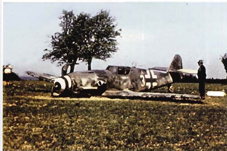
ABOVE: 'White 3', a late production Bf 109 – either a G-10 or a G-14/AS belonging to the 1. Staffel of an unidentified Jagdgeschwader – one of two that crash-landed behind Allied lines at the end of the war. The camouflage was 83/75/76, with a soft-sprayed application of 02 over the side surfaces to tone down the 76-colouring. The 'yellow' elevator was, in fact, just the yellowish-muddy spray that had been thrown up during the belly-landing. The Balkenkreuz and Hakenkreuz markings were of correct style. The presence of just a spiral spinner marking, and no yellow tactical markings, indicates that the aircraft had been serving with a unit on the Western Front, yet it lacked any Reichsverteidigung band markings, something that became more frequent in the closing weeks of the war. (J. Crow)
