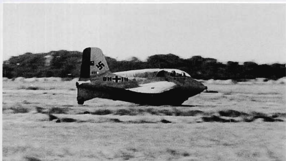
RIGHT: The prototype aircraft of the Me 163 B series retained their overall 76-finish until August 1944, by which time camouflage was considered essential. Seen here is the V 35, W.Nr. 163 10044, GH+IN. The rudder was a replacement, still in dark red-brown fabric primer.
