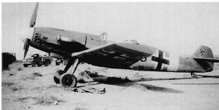
ABOVE: Once the RLM had standardised its tropical colours, two forms of factory standard application followed. One was a solid application of 79 on all upper and side surfaces with 78 lower surfaces as seen here on Lt. Mix's Bf 109 F-4 trop of 6. Staffel, II./JG 27, shot down near El Alamein on 14 August 1942. Note the increased size of the Balkenkreuz, a locally applied variation common to Bf 109s and Bf 110s in the final stages of the North African campaign. A full complement of white tactical markings was by then in use. (D. Vincent)
