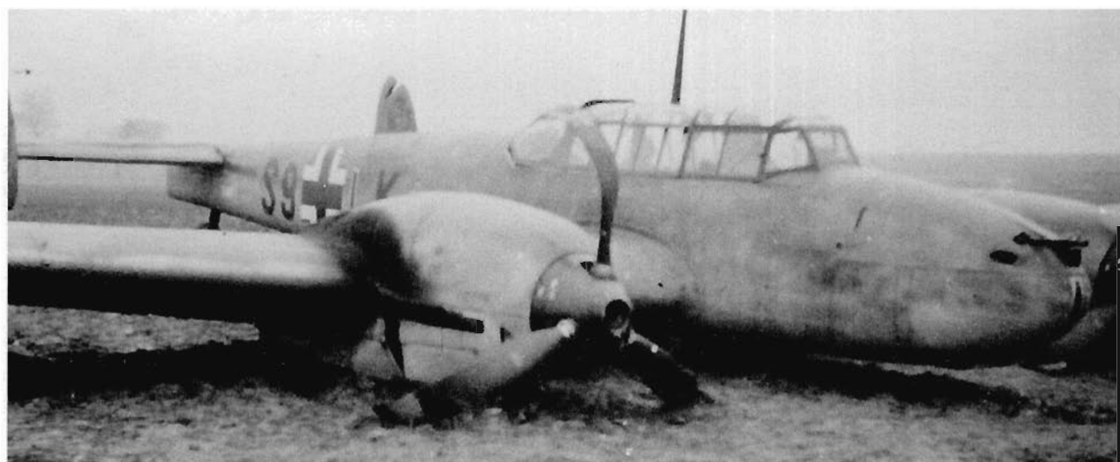
ABOVE AND LEFT: Uffz. Artez' Bf 110 D, S9+LK, of 2./Erprobungsgruppe 210 photographed after a forced-landing on 21 March 1941, following a night bombing attack. Camouflage was still 71/02/65 with a thin spray of 02 over the camouflage of the fuselage and engines. The extended tail cone housed a dinghy. (J.Vasco)
