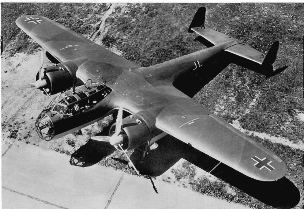
BELOW: A Do 17 Z-1 wearing the regulation standard factory finish 70/71/65 scheme of 1938. The main stencil markings on the wings were in yellow. Application of the pattern conforms completely to the RLM standard.
