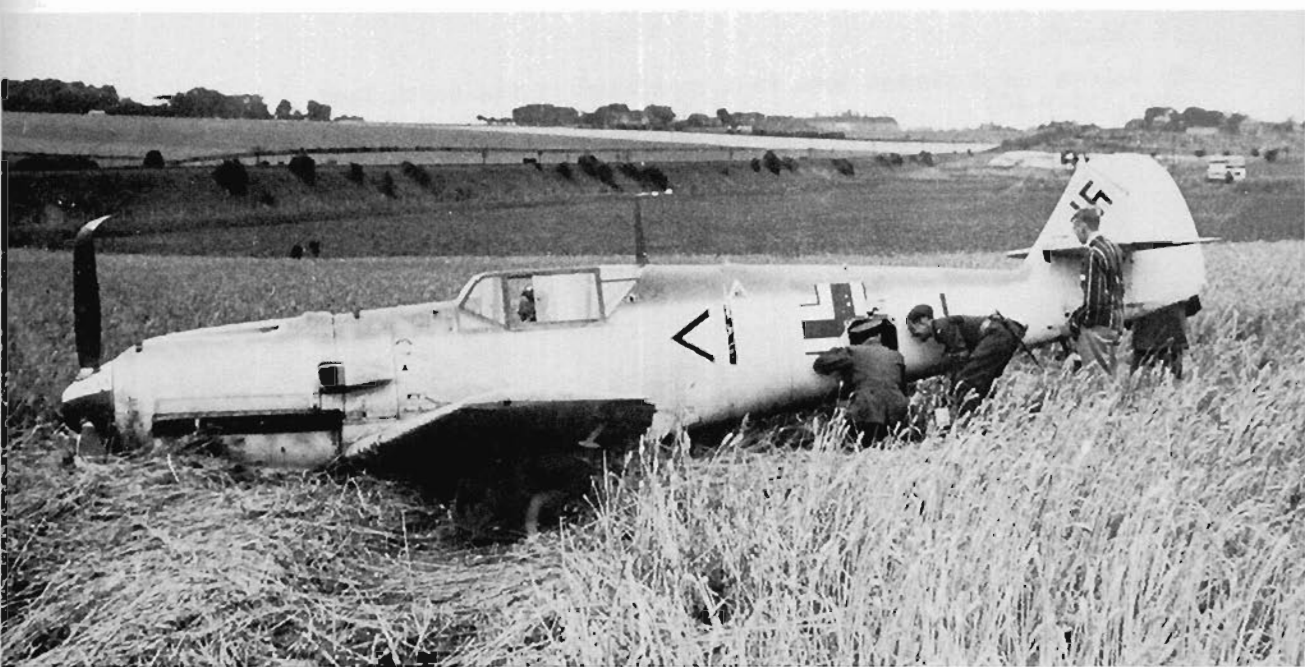
ABOVE AND RIGHT: Oblt. Werner Bartel's Bf 109 E-1, W.Nr. 6296F from the Stab of III./JG 26, brought down on 24 July 1940, displayed the first tentative changes to the camouflage revisions that had been introduced at the end of 1939. Upper surfaces were 71/02 but with transition to the 65-sides applied with a soft sprayed application along the engine cowling to produce a ragged effect. Very soft traces of mottling, in both colours, had been added to the engine cowling, down to below the exhaust stubs. The gun troughs were a pale colour, something still seen fairly often at that period of the war. Judging from other photographs, the colour was probably 65, not yellow or white as has sometimes been suggested. Note the tonal contrast between the 70 of the propeller blades and the darkest upper surface colouring. The spinner was black with a one-third white segment, another recently introduced change to fighter aircraft. The suffix 'F' (Flugklar) to the Werknummer indicated that it was a repaired aircraft (apparently also upgraded from original E-1 configuration, probably at the same time), which probably accounts for the additional camouflage revision. This form of suffix to the Werknummer did not continue much beyond this date as the Luftwaffe revised its system of repair codes and symbols. The illusion of a very pale rudder colour was produced by the angle of the rudder to the sun, something confirmed from the head-on view.
