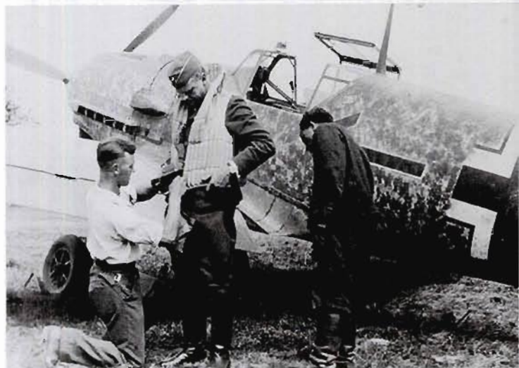
BELOW: This view of a Bf 109 E-3 of Oberstleutnant Harry von Bulow-Bothkamp, Geschwaderkommodore of JG 2, provides a more detailed example of the stippling style of application that illustrates that brushes were used, not sponges. Note the overlapping of the edges of the Balkenkreuz with the 71-colour, which was confined to the 65-coloured areas of the fuselage side surfaces. (E. Mombeek)
